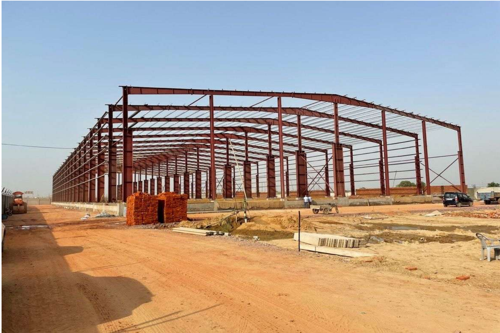
Warehouse Shed, Uttarakhand
